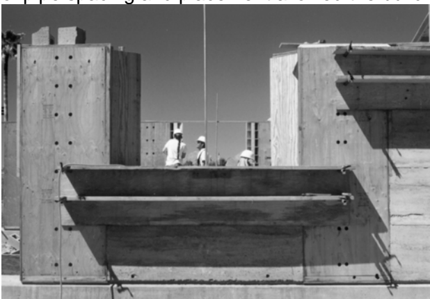
Figure 2. Incremental rammed earth forms assembled using simple elements.
