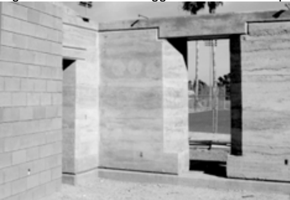
Figure 4. Rammed earth walls completed.
