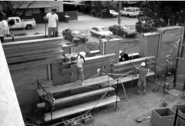
Figure 3. Forms are staggered to allow tamping at several locations simultaneously.
